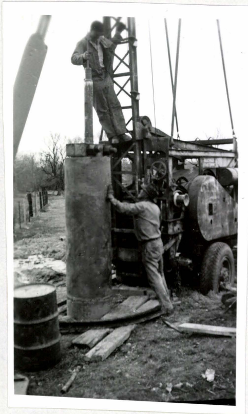
Fig. 25A Driving Head on the 24-inch Casing
