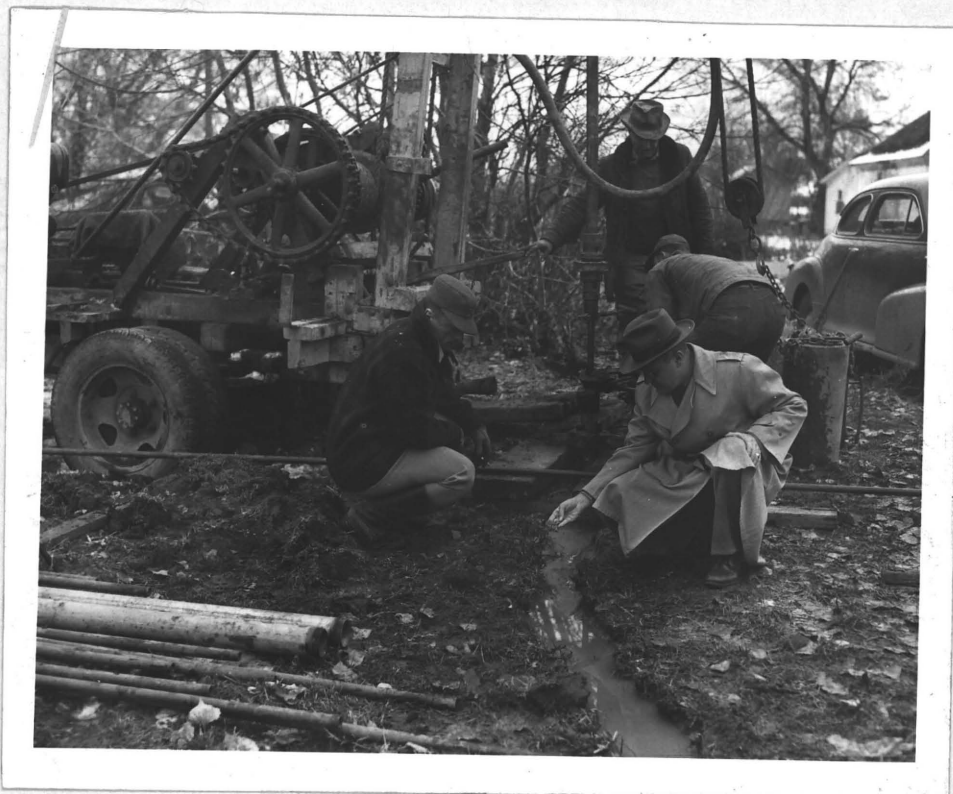
Fig. 10 Examining Material at Test Well No. 2
