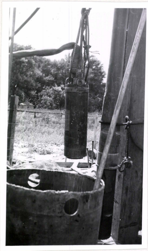
Fig. 22 Submersible Pump Ready to be Lowered into Well No. 3
