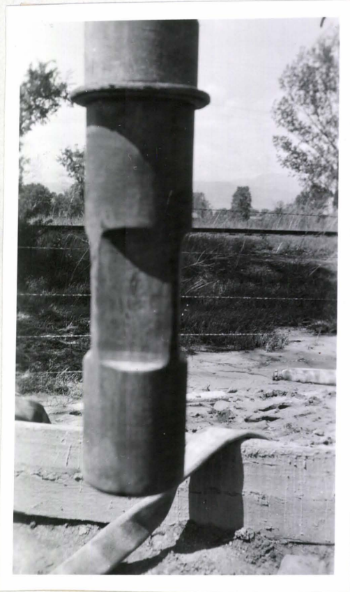
Fig. 28 Surge Block Used for Developing Well
