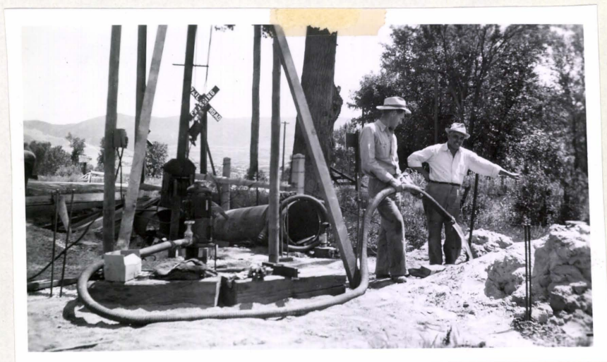
Fig. 33B Testing New Turbine Pump
