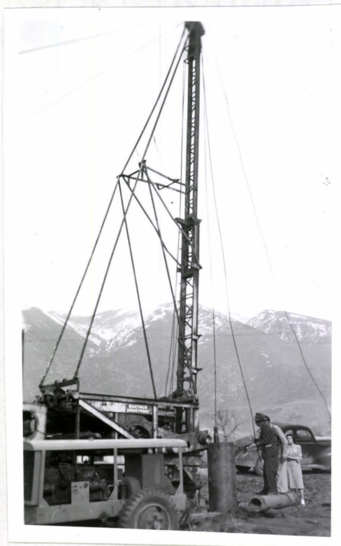
Fig. 26 Drilling in Progress
