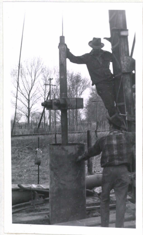
Fig. 25B Driving Head Ready to Drop
