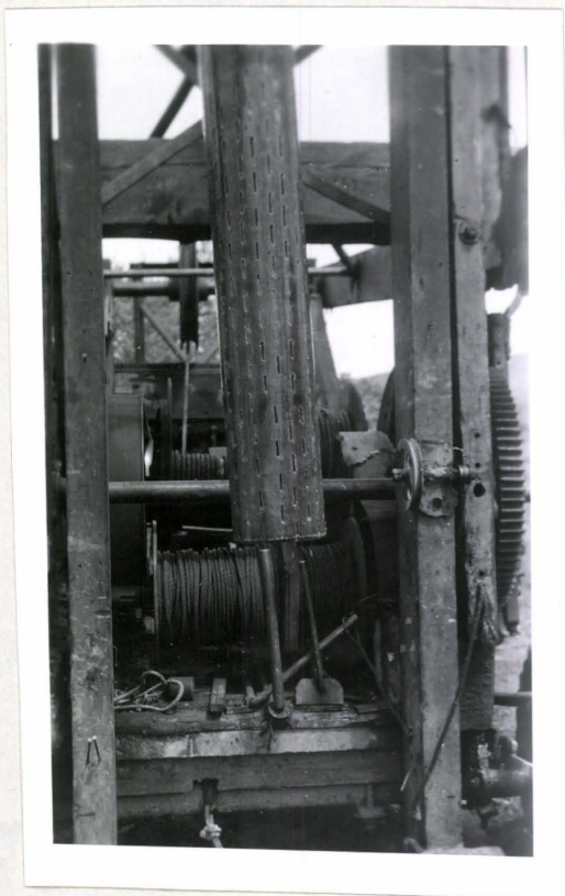
Fig. 19 Perforated 8-inch Casing Showing Perforations and Plate Welded at Bottom
