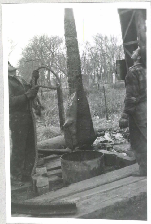
Fig. 23A The 20-inch Bit Being Raised From Well
