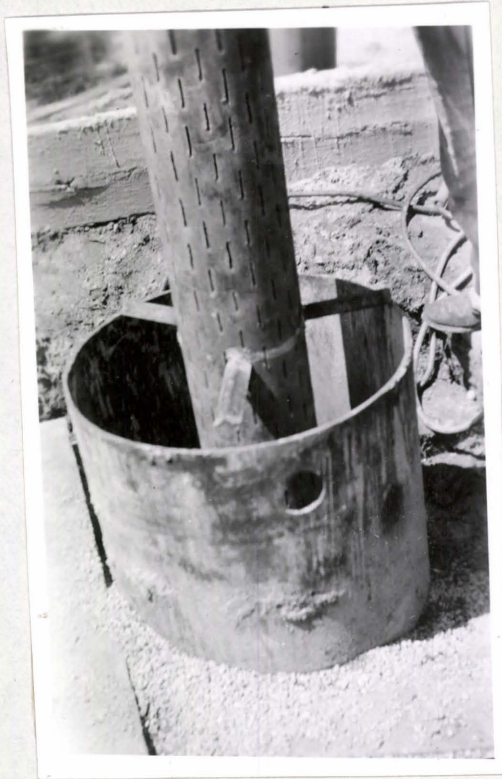
Fig. 18 Spacers Welded to 8-inch Casing
