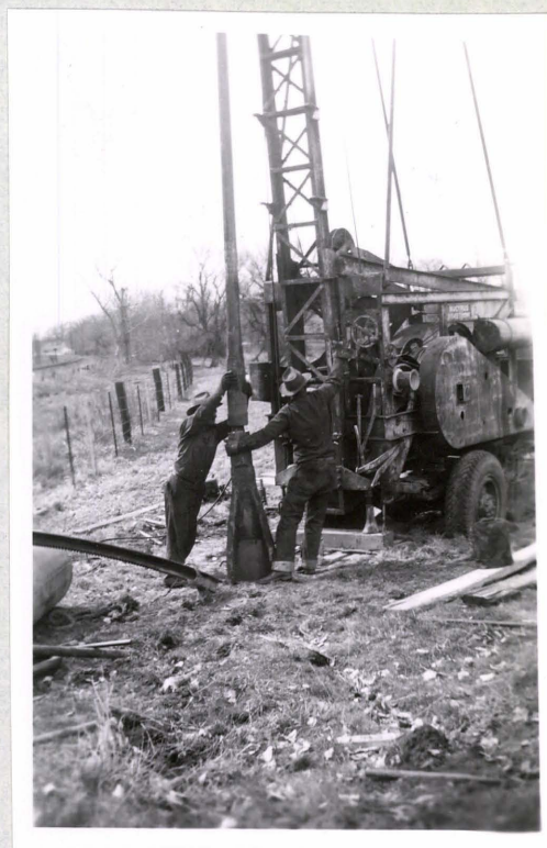
Fig. 23B The 20-inch Bit Being Connected to Drilling Tool
