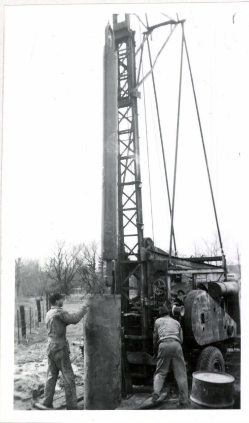
Fig. 24A Bailer Being Raised From Well
