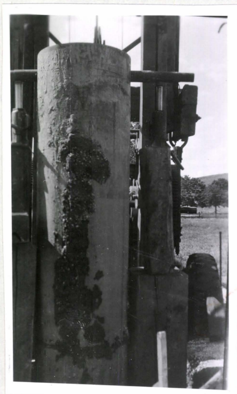
Fig. 27 Jacking Back 24-inch Casing
