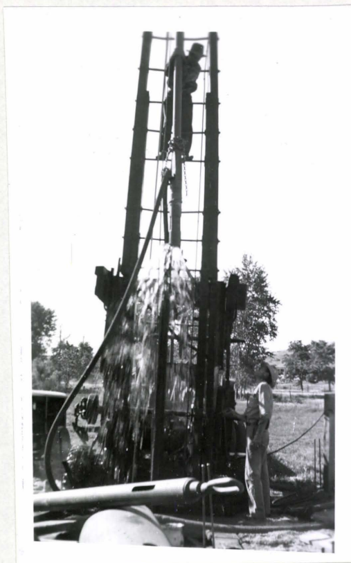
Fig. 29 Installing the 5-inch Pilot Tube by Jetting and Driving
