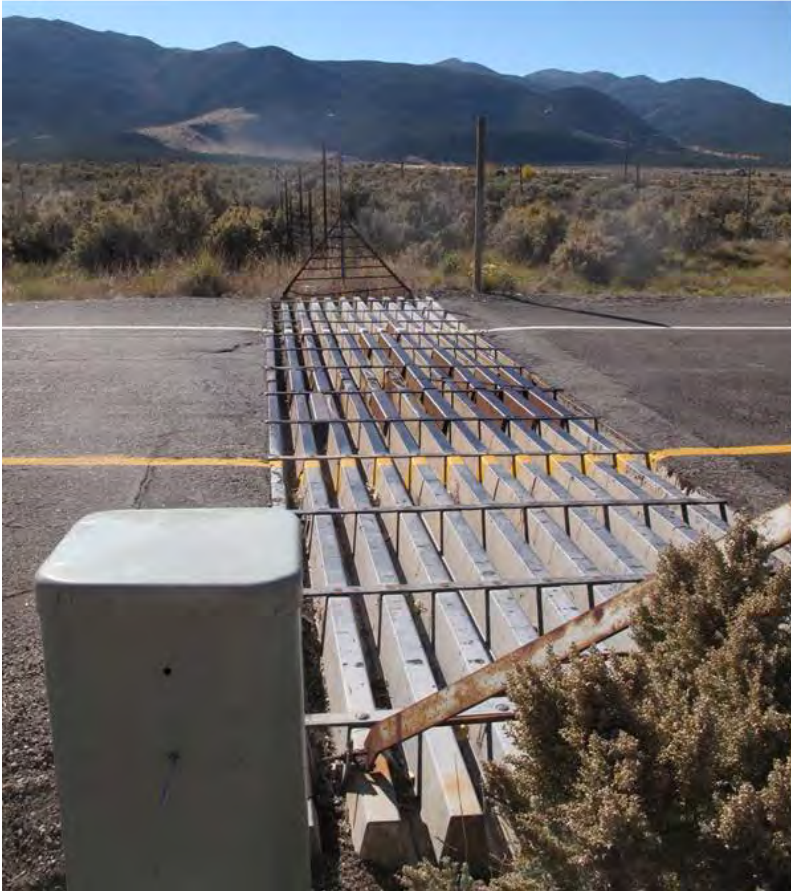
Figure 2. Cattle guard (1.9-m \times 9.7-m) not constructed over excavation (A) and close view of cattle guard rails (B) on an access road to Interstate 15, near Summit, Utah, USA.
