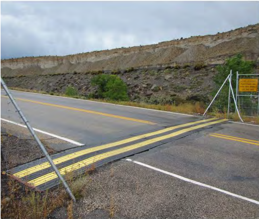
Figure 6. Electrified mat (1.2-m × 11-m, A) and close view of composite planks with embedded metal electrodes (B) on an access road to U.S. Highway 6, near Helper, Utah, USA.
