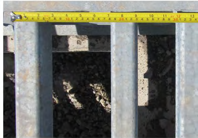
Figure 4. Double cattle guard (4.6-m \times 7-m) suspended over excavation (A) and close view of cattle guard rails (B) on an access road to U.S. Highway 91, north of Mantua, Utah, USA.
