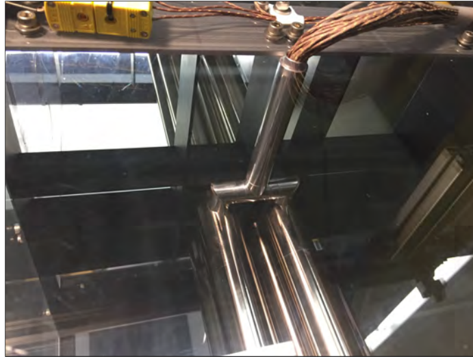
Fig. 3.8: Close-up of the conduit used to route thermocouple wires from the rod centers to the data acquisition system outside the test section.
