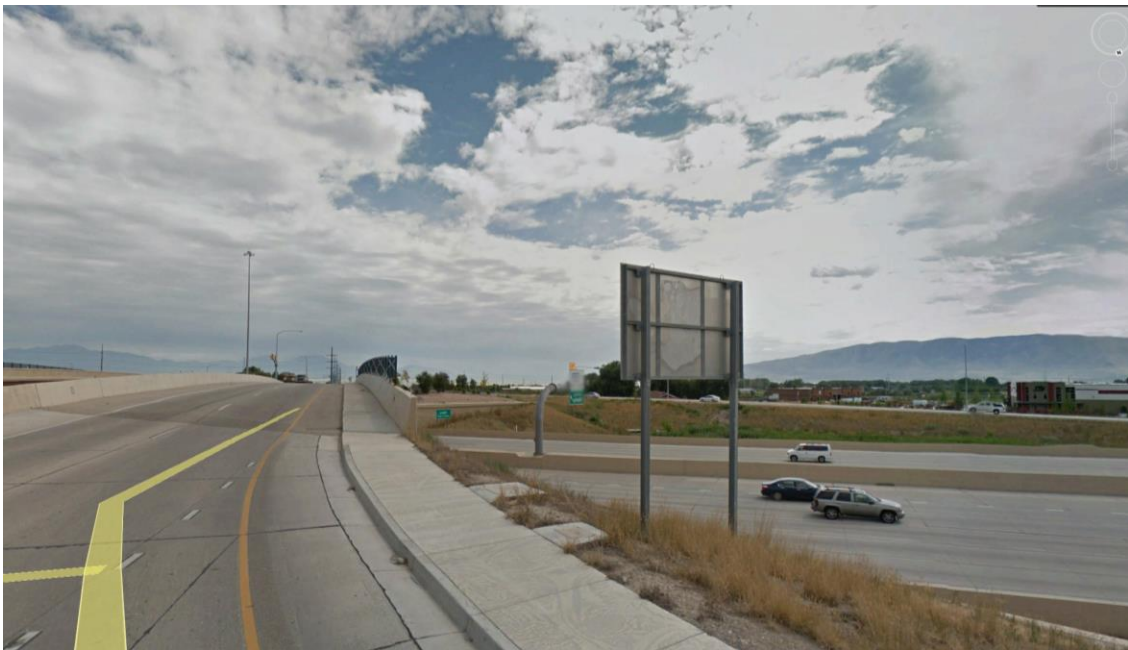
Figure 12 American Fork Main Street (Exit 278) DDI Outside Walkway (Google Maps).
