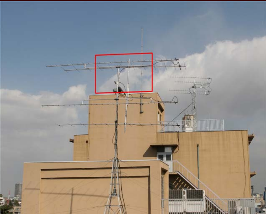
ISSL station (under construction)
