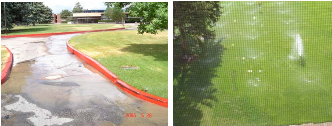
Figure 3 Water is frequently wasted from traditional high water use landscapes due to faulty sprinkler heads or poor irrigation design contributing to excessive water use and runoff.
