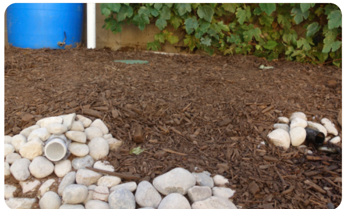
A backyard in Albuquerque, NM, with both a shower greywater outlet (black) and rain barrel overflow (white). Credit - Roslynn Brain
