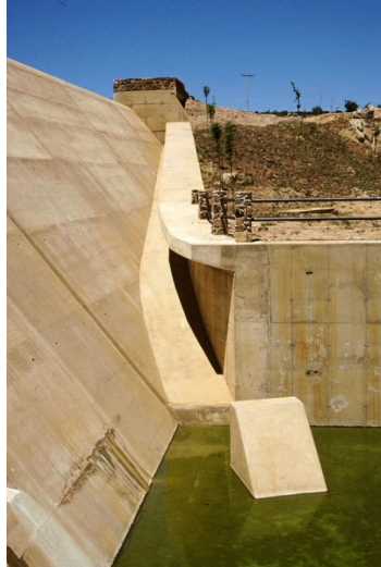
Figure 5. Picture of an impact block in the HCC spillway in Zapardiel de la Cañada Dam (Spain).
