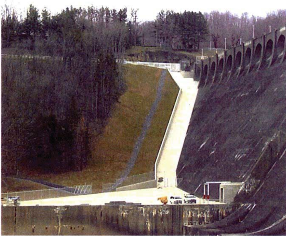
Figure 2. Overtopping protection of the right abutment of Tygart Dam (USA) (FEMA 2014).
