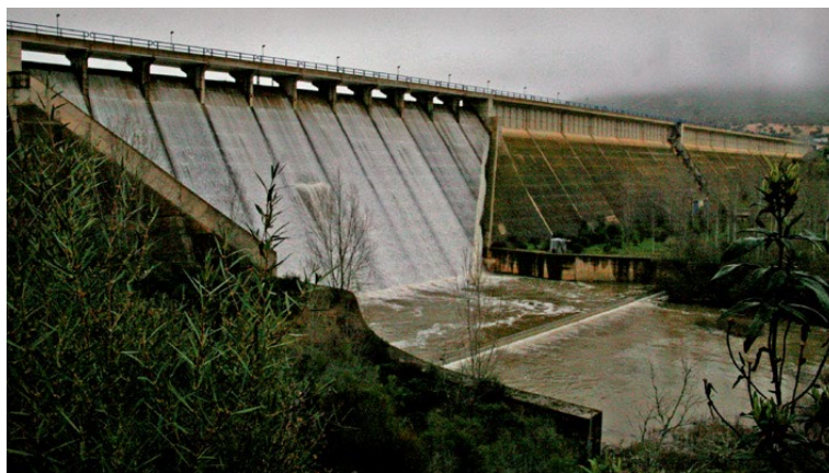
Figure 1. Spillway of the Torre de Abraham Dam (Spain) in operation.
