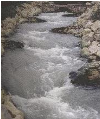
Figure 1. Natural Bypass Channel for Salmon in Loue River
