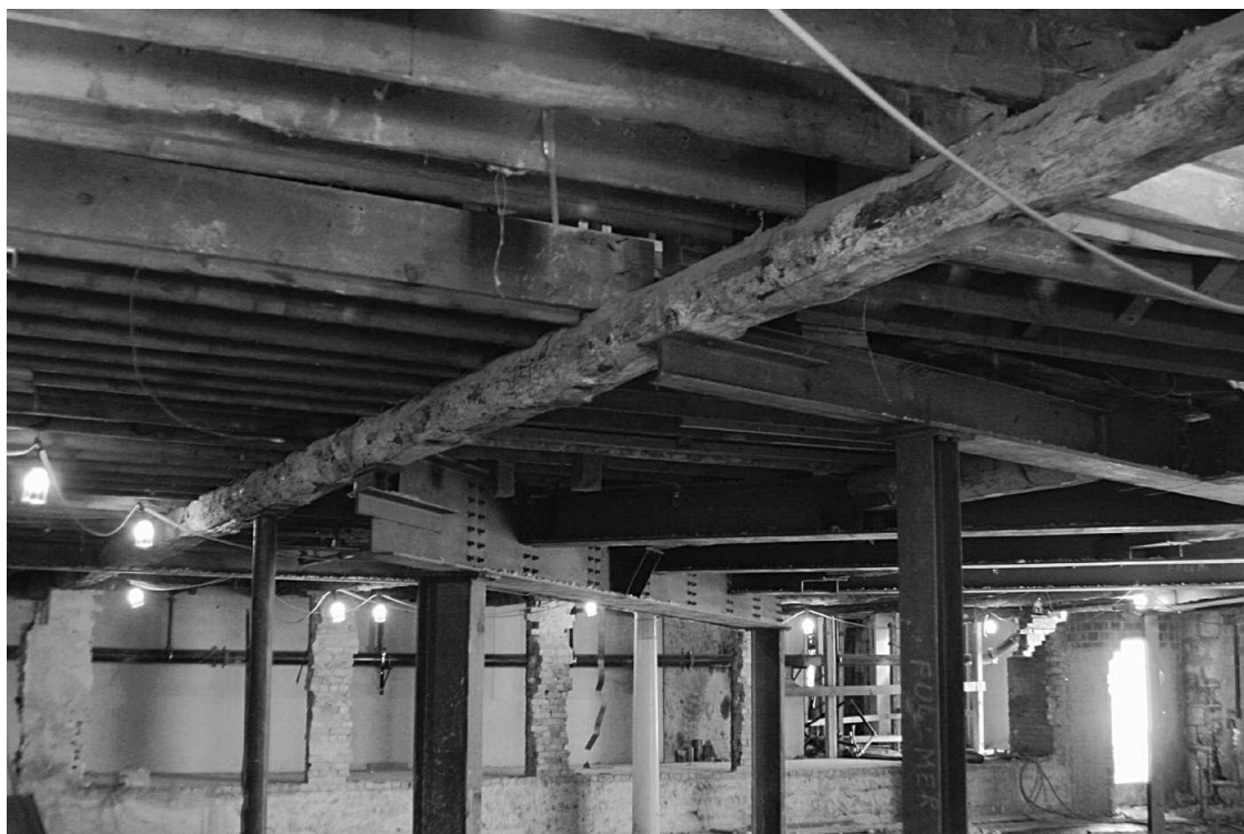
Figure 3. Interior of the Salt Lake Tabernacle underneath the main level, showing original timbers and brick piers (background), along with steel beams from previous renovations.
