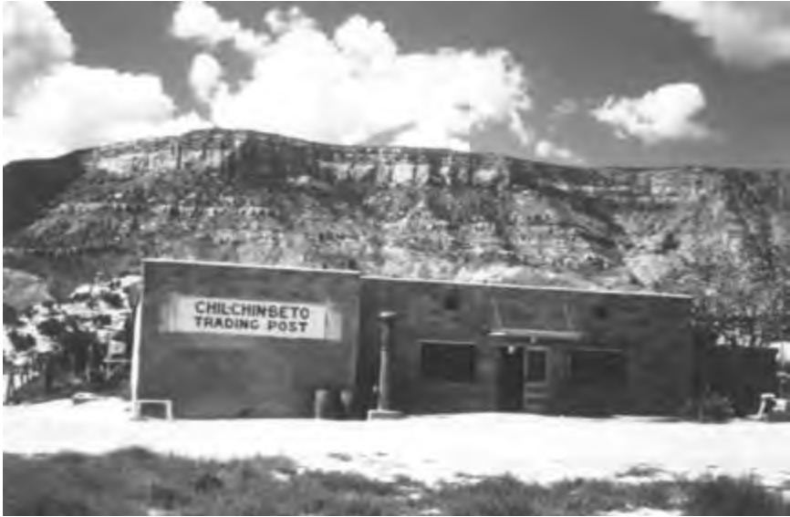
Chilchinbeto Trading Post in 1956. The left side of the structure was the original post, while the right side is an addition made in 1944. Behind the post sits Black Mountain. (Photo by Joe C. Hunt)
