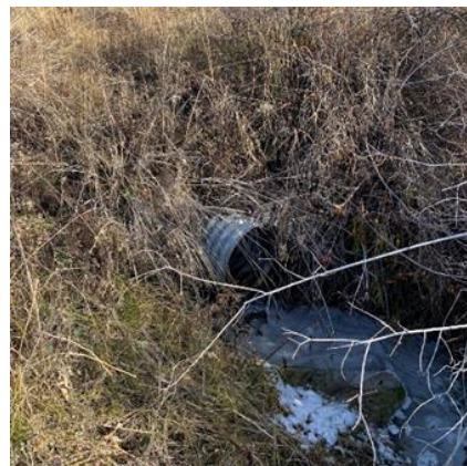
Figure 32. Photo of culvert on the Porcupine Creek.
