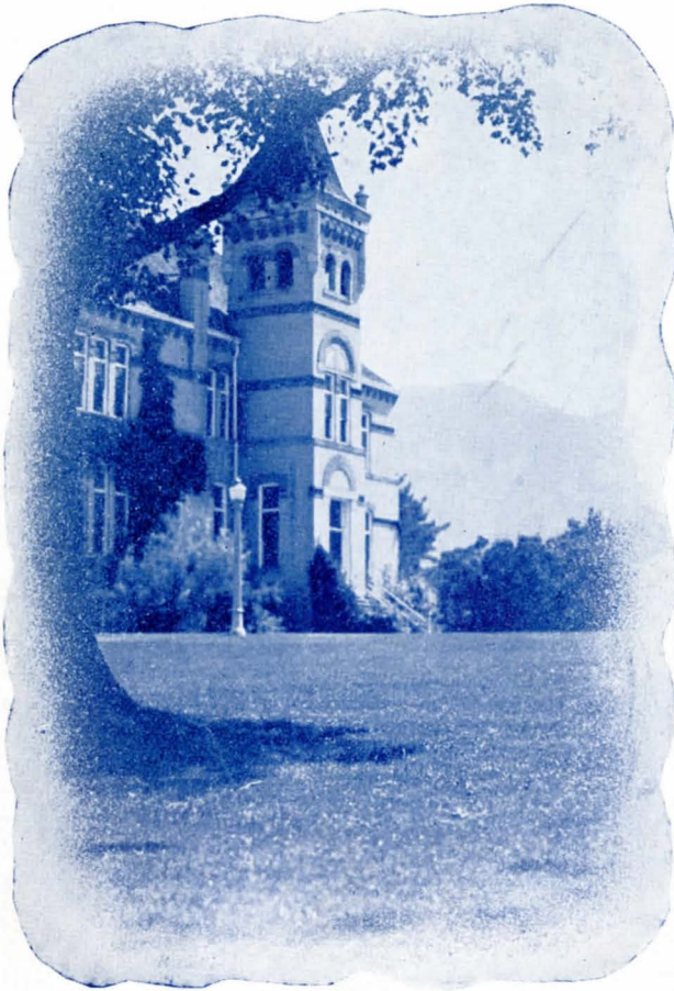
South Wing of Main Building where cornerstone slab will be opened for first time in 50 years, March 8, 1938.
