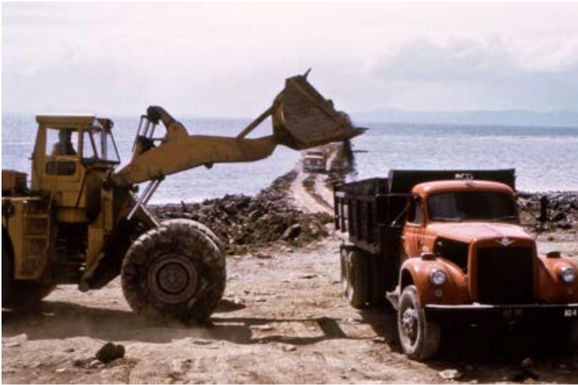
Figure 14. Construction image of Robert Smithson's Spiral Jetty (1970)
