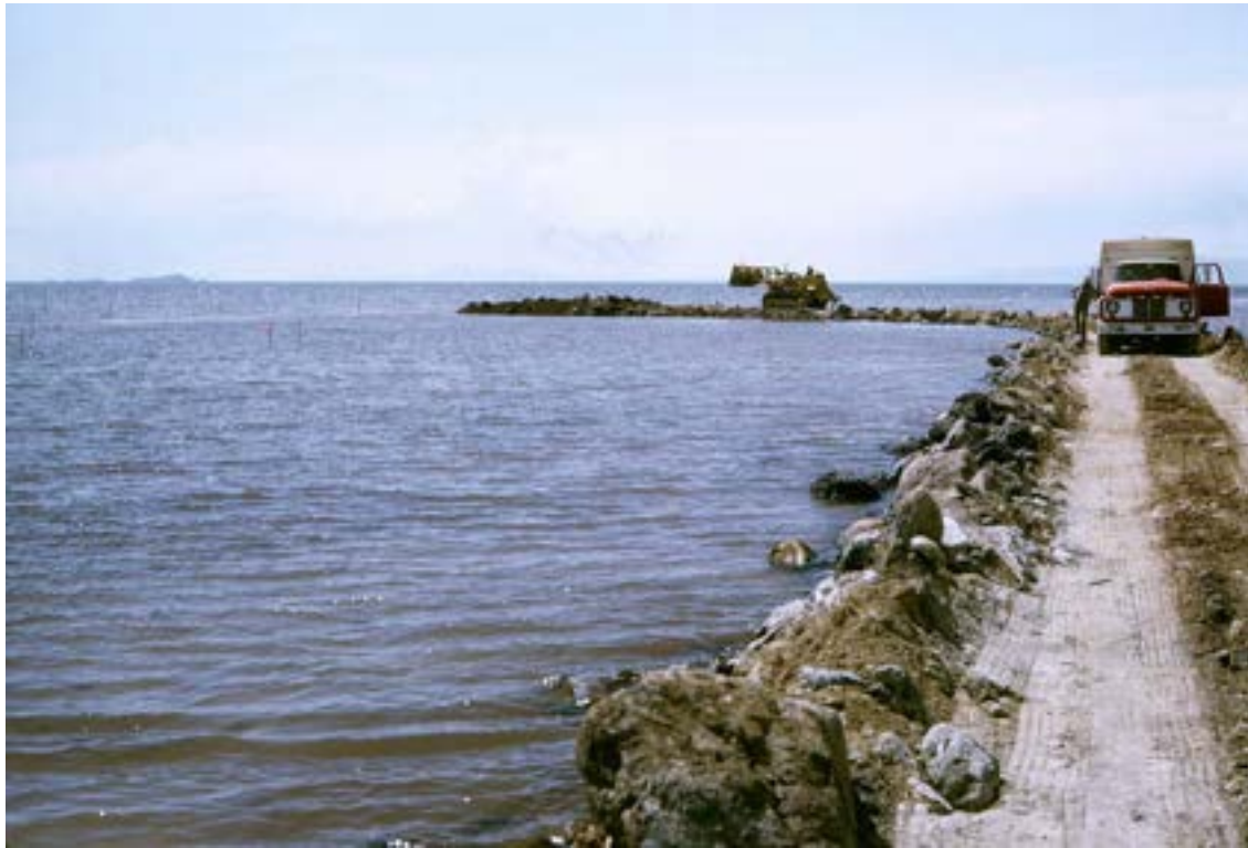
Figure 15. Construction image of Robert Smithson's Spiral Jetty (1970)
