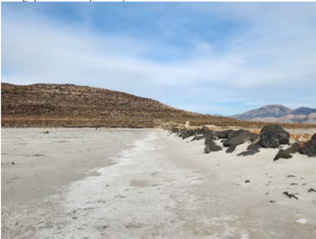
Photograph 13. Tail of Spiral Jetty showing slope from earthwork to lakebed. Camera view east.
