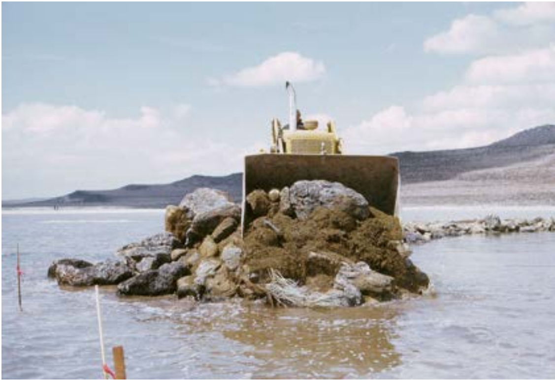
Figure 16. Construction image of Robert Smithson's Spiral Jetty (1970)
