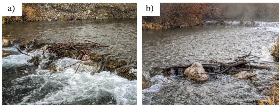
Figure 6 – Stream-wise and channel-spanning LWD entrapped at a BSF River rock weir October 29, 2021 (photo courtesy of K. Margetts).
