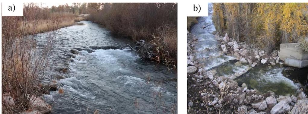
Figure 1 – Examples of rock weirs including a) a V-Notch rock weir located in Blacksmith Fork River, Hyrum, Utah, USA (photo courtesy of K. Margetts) and b) a rock ramp acting as a natural fish ladder in Rock Creek, Montana, USA (photo courtesy G. Jordan).
