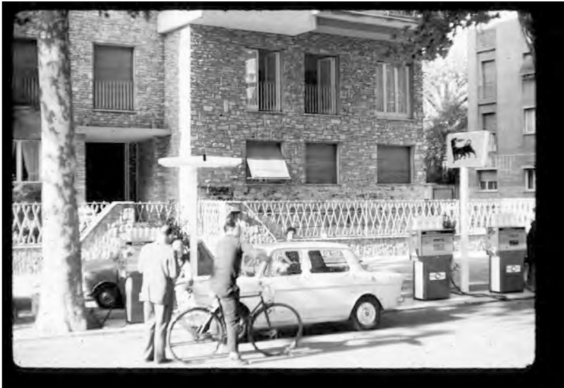
The mission office at Viale Mazzini 35 in Florence which by summer 1967 had replaced the original headquarters at Via degli Artisti 8. Photo courtesy of Noel Zaugg.
