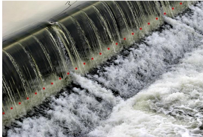
Figure 6. Aggregation of a significant water cushion (red dotted line) at the weir Auxonne (France)
