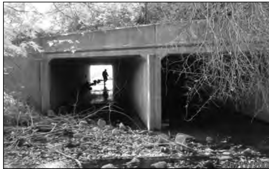
Figure 1. Large double culvert.
