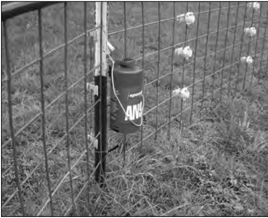
Figure 2. An electric fence charger was attached near a T-post and on a panel that is curved to the outside, requiring additional insulators to keep the wires from grounding out to the fence.
