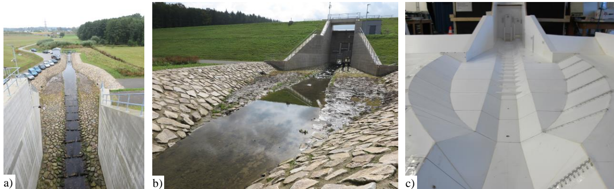
Figure 3. FRB Neuwürschnitz, Saxony: a) dam downstream side with ecological culvert, pass channel and DSSB; b) DSSB and ecological culvert; c) DSSB physical model test.
