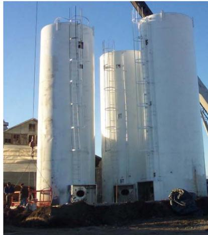
Figure 2-6. Induced Blanket Reactors (IBR) under construction.
