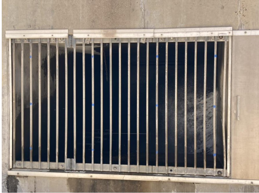
Figure 2 Air grate at energy dissipating structure.
