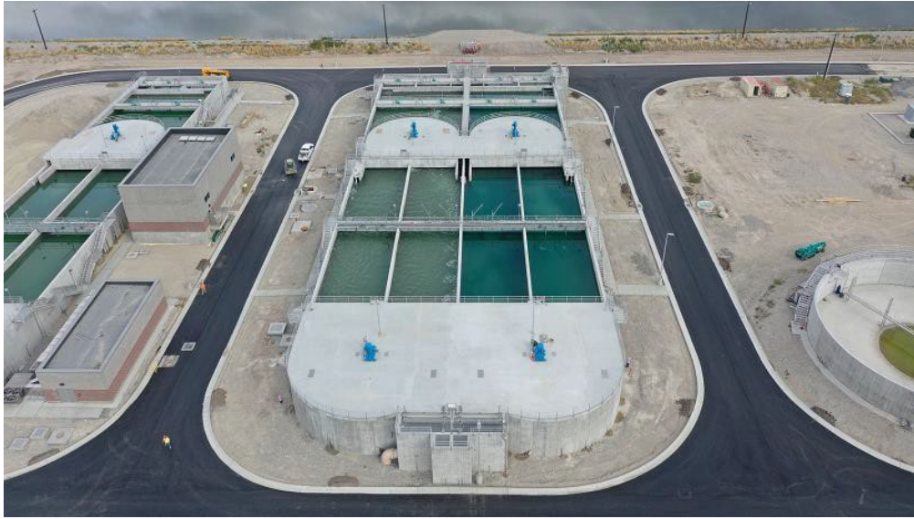
Fig. 10. Bioretention basins at the Bardenpho Plant
