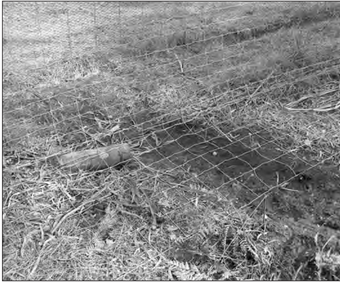
Figure 1. Wire mesh (hinge-joint wire) stretched flat across the ground and attached to the existing deer fence.
