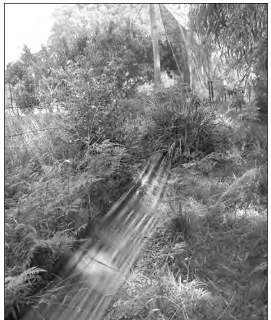
Figure 2. Flexible woven material (silt fence) attached to existing deer fence and secured to the ground using tent pegs.
