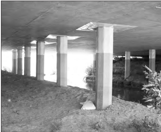
Figure 3. Highway structure with PTFE surface modification.
