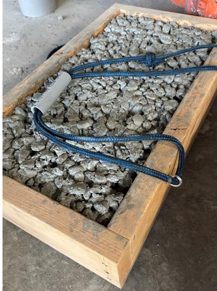
Figure 3-7: Handles attached to forms
