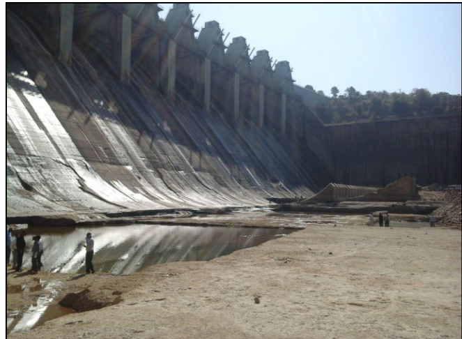
Photo 2. The eroded apron of bucket
