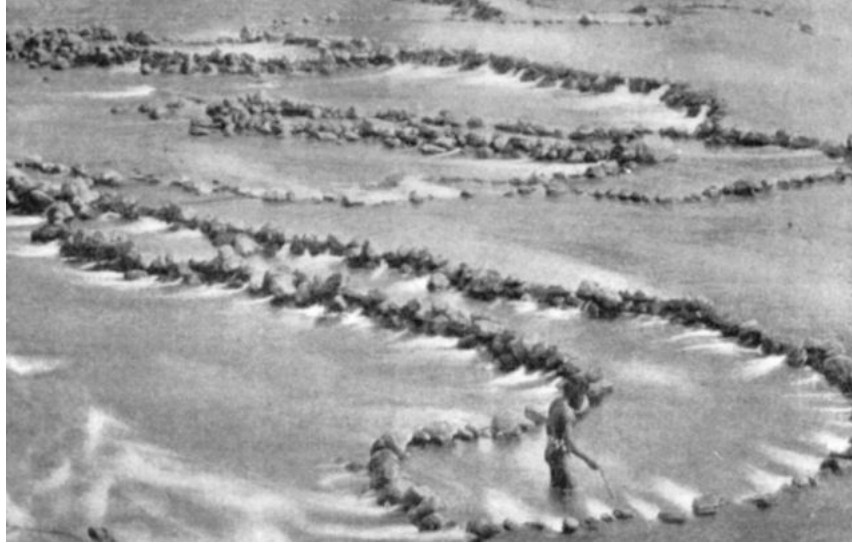
Figure 1. Historic (probably posed) photo of a man fishing in the Brewarrina Aboriginal rock fish traps / Baiame's Ngunnhu, published in The Dawn 1893 - Main flow direction from bottom right to top left.
