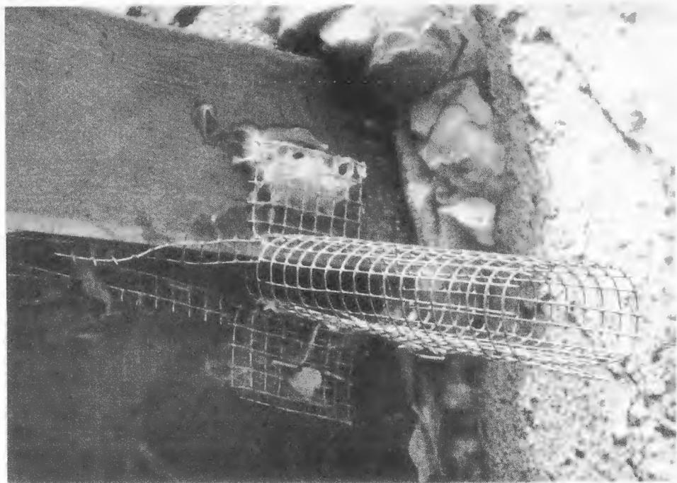
Figure 5. The Hanks' excluder device is a hardware cloth oval cylinder that extends the opening of the roost away from the building. The dimensions of the device are dictated by the species of bat being evicted.
