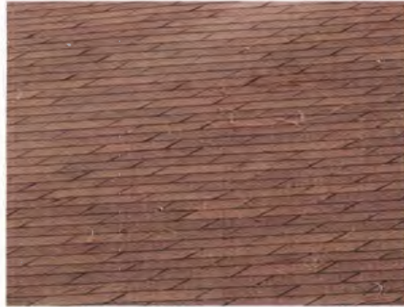
Heavy asphalt shingles
