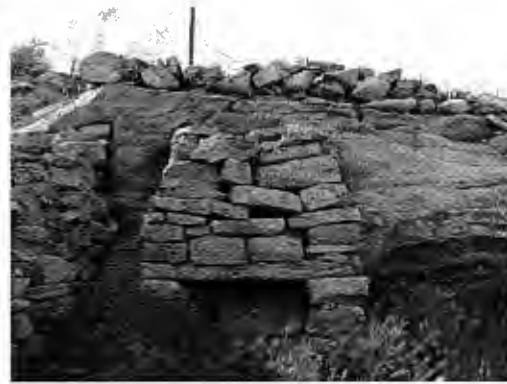
Figure 3.4 - Fireplace in Dwelling
