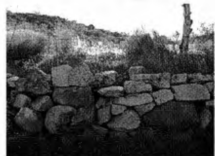
Figure 2.10 - Rock Retaining Wall
