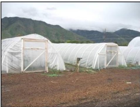
Image 1. High tunnel constructed with PVC and wood frame.
