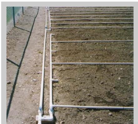
Main distribution lines are glued, lateral lines are not glued
