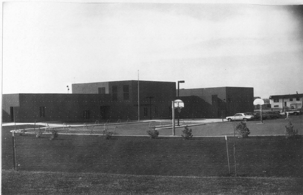
Photo 7. West Elementary School.
