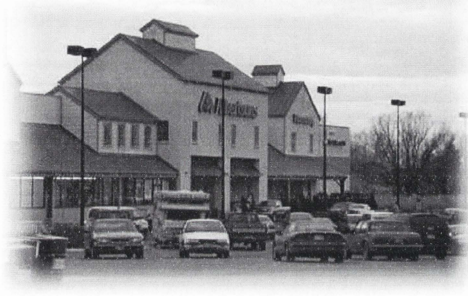
Figure 29. Albertson's Agricultural Theme Commercial Complex – Lehi, Utah
