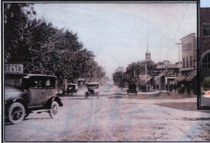
Main Street, note the power poles moved to the side, ne Clark Collection.
