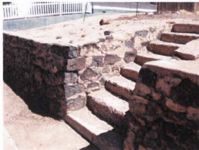
An existing basalt rock wall offset 2' from the sidewalk and less than 4' tall.
