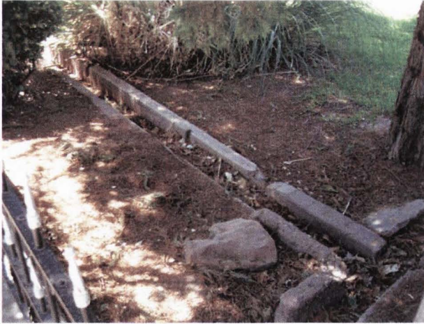
Fig. 14 Existing residential irrigation ditch lined with concrete and stones.
