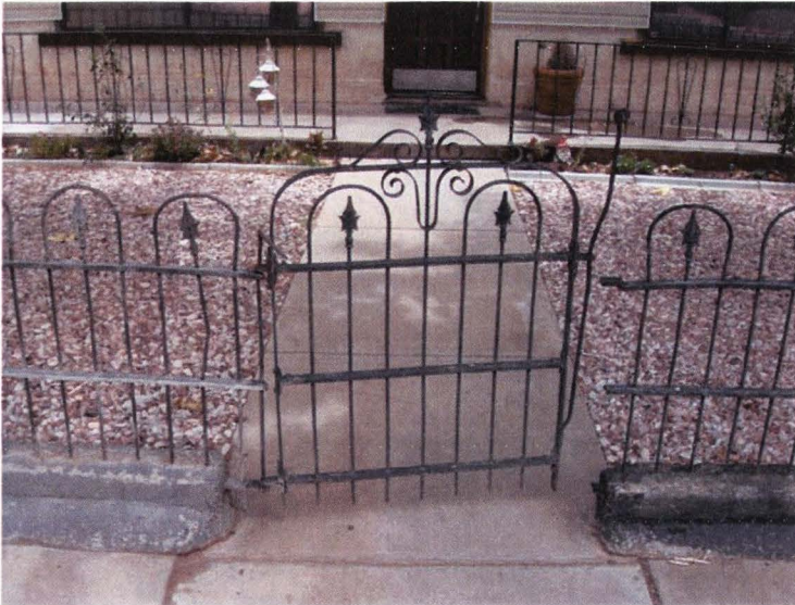
Fig. 27 An existing wrought iron fence similar to the ones seen in historical photographs. This fence shows the bow and picket style fence with the scalloped picket.
