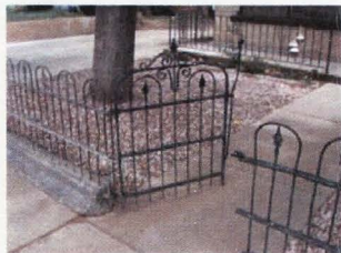
An original wrought iron fence located in front of a residence in St. George, showing the bow and picket style.
