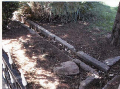
Remnants of a residential ditch at the Whitehead Home near the Seven Wives Inn.
