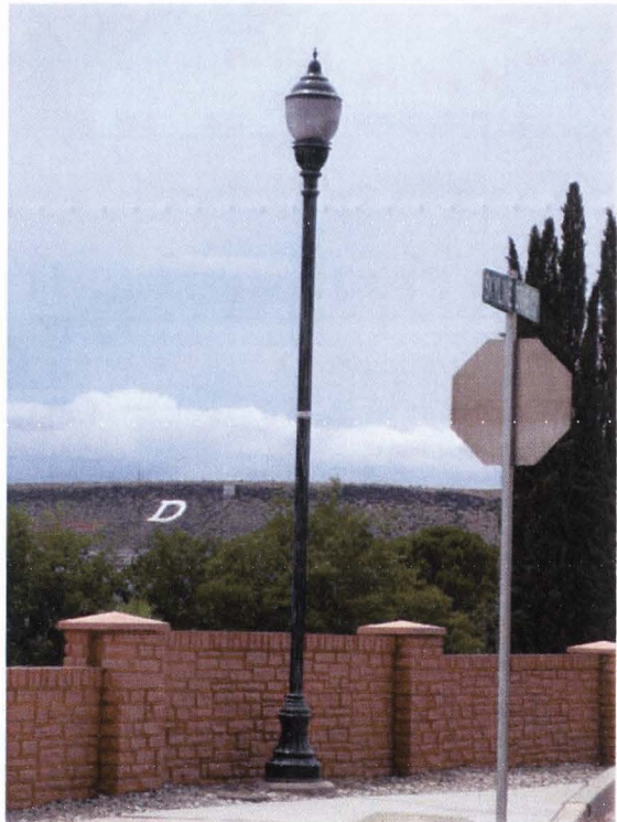
Fig. 23 One of the many street lamps used in the historic downtown. The dark metal night-friendly cap is used on the top half of the globe. This image also shows the correct Cooper Lighting post with the exception of color (2007).
