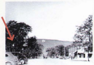
In 1930-40s Tabernacle Street maintained the same lamp post fixture and location as in the 1920s.
