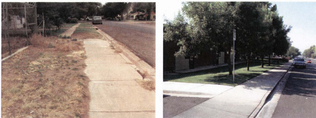
Fig. 6 These images illustrate the inconsistent treatment of the planting strip. In the image on the left, an integrated sidewalk and curb/gutter leads right into a turf planting strip. The image on the right shows trees planted on the inside of the sidewalk eliminating the planting strip.
