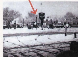
The lamp post to the left of the PEP sign is similar to all the previous lamp posts. This photograph was taken between 1933 and 1935.
