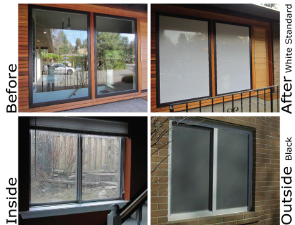
Figure 4. Various patterned films designed to prevent bird window collisions. Films are transparent on one side and reflective on the other. Photos courtesy of Collidescape.
