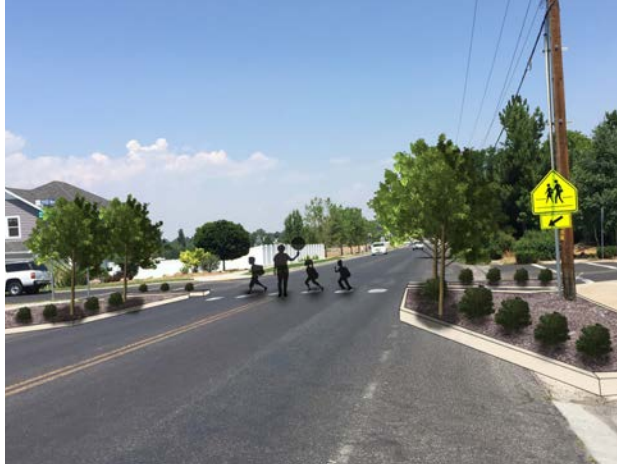
North Park Elementary improved school crossing with curb bulb-outs to minimize crossing width and to slow traffic.
