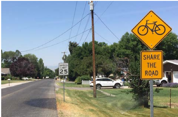
3C Signed Shared Roadway (2200 N./1200 E.)
