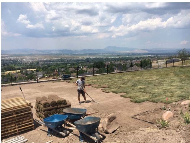
Figure 2. Soil preparation prior to sodding (photo credit: Grant Cardon).
