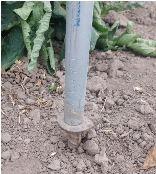
Figure 2. Metal conduit piping over rebar pounded into the ground. A washer, welded onto the rebar to prevent conduit from sinking into the soil.
