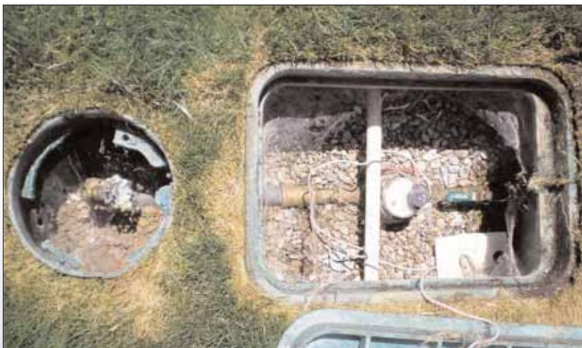
A standard secondary connection like this one involves a simple configuration of a meter and valves.
