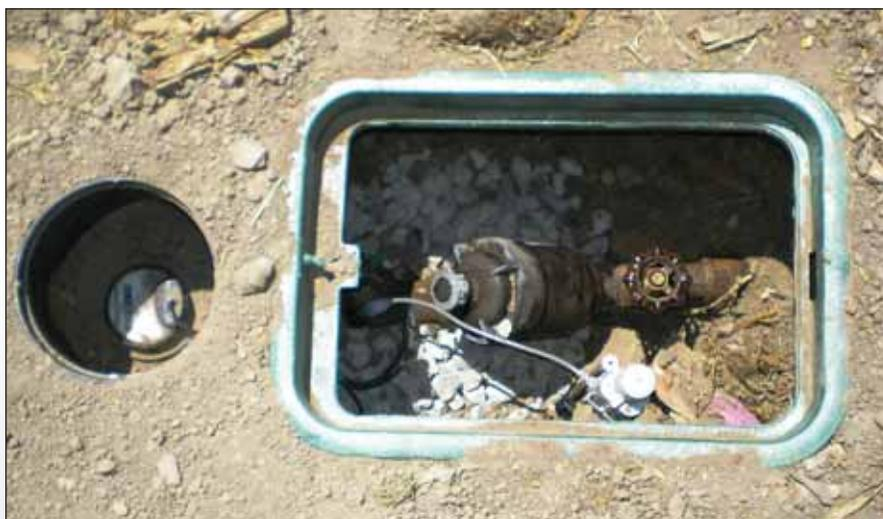
A standard secondary connection such as this one consists of a valve, filter, drain, and meter contained in one or two valve boxes.
