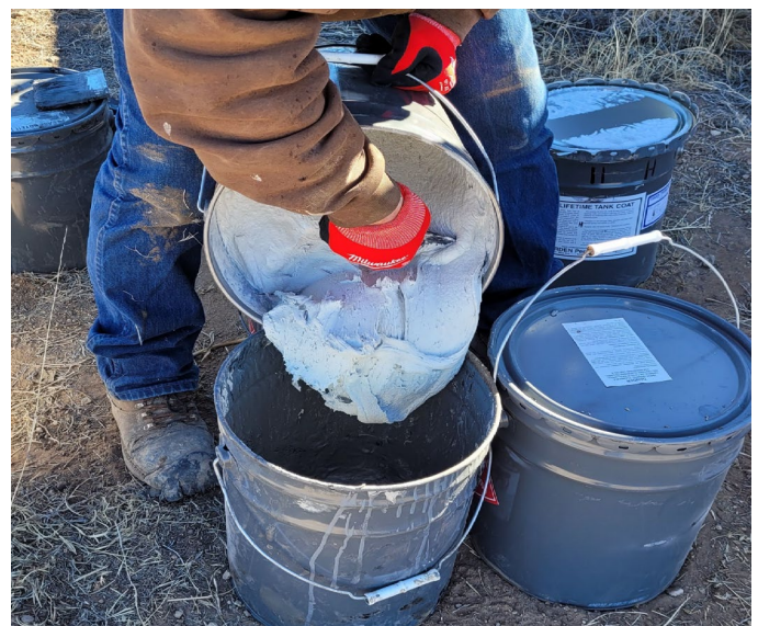
Figure 3. Mix Epoxy Resin and Hardener in Equal Parts
