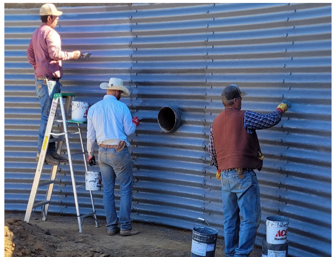
Figure 5. After Application, Wait 24 Hours and Apply a Second Coat of Epoxy
