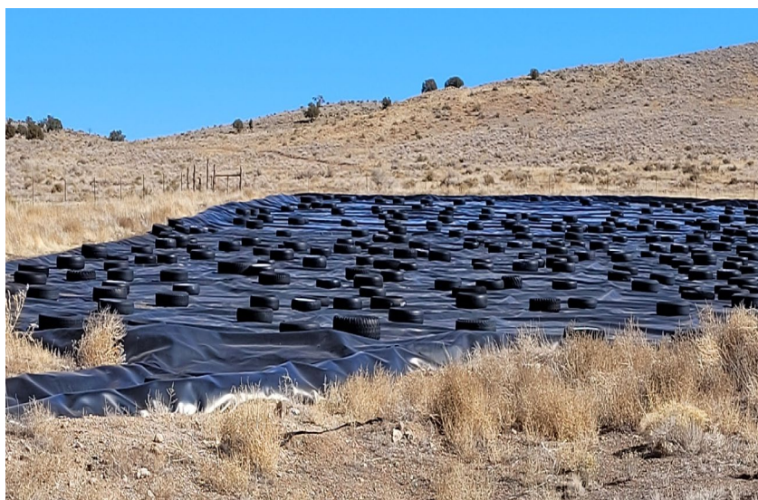
Figure 1. Rubber Water Catchment Apron Anchored With Used Tires
