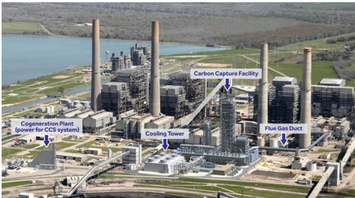
Figure 2. Petra Nova Is a Coal-Fired Power Plant With Carbon Capture and Storage (CCS) Near Houston, Texas
