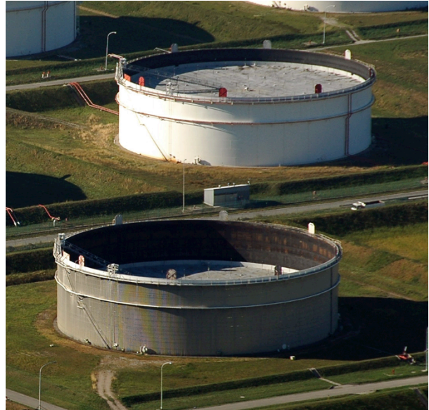
Figure 4: Floating Roof Oil Tanks
