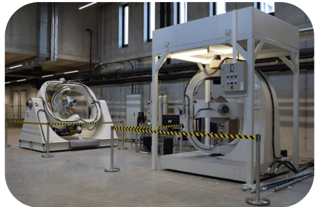
Figure 6: Dynamic Bench Test Facility at ZfT premises for three-axis satellite motion simulation
