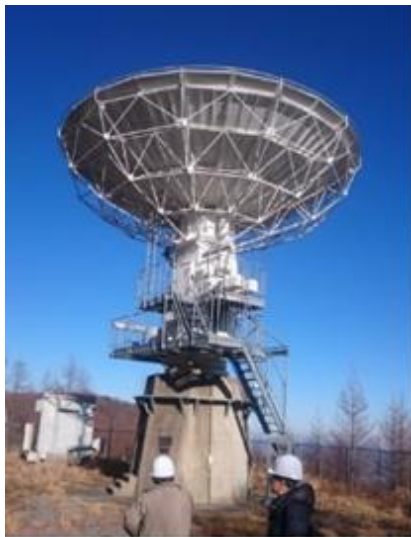
Fig.7 10m X band dual polarization Antenna at Usuda Deep Station, JAXA, Japan.
