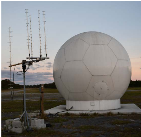
Figure 2: MLB MC3 Node – UHF Yagis and S-band Dish/ Radome
