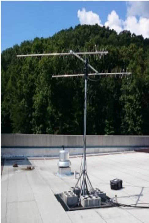
Figure 3: UHF –VHF Cube Satellite Ground Station
