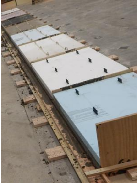
Figure 3-15 Completed first wythes with foam and connectors in place
