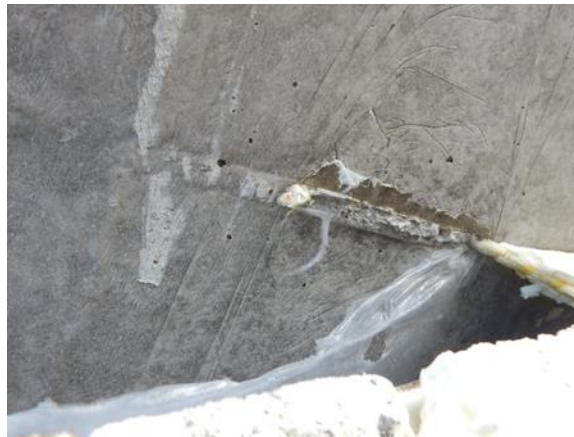
Figure 4-19 Shear fracture failure in unbonded specimen with EPS foam
