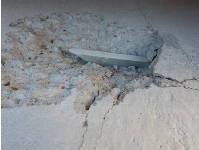
Figure 4-31 Punch through close-up
