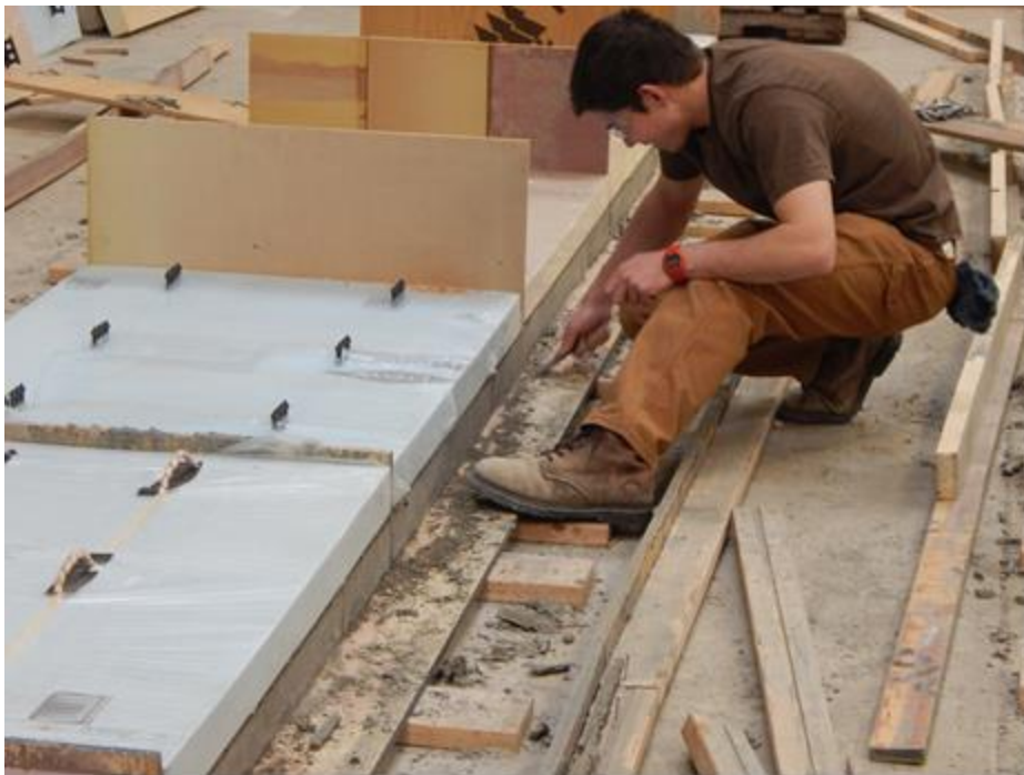
Figure 3-16 Clean-up following formwork removal of first wythe
