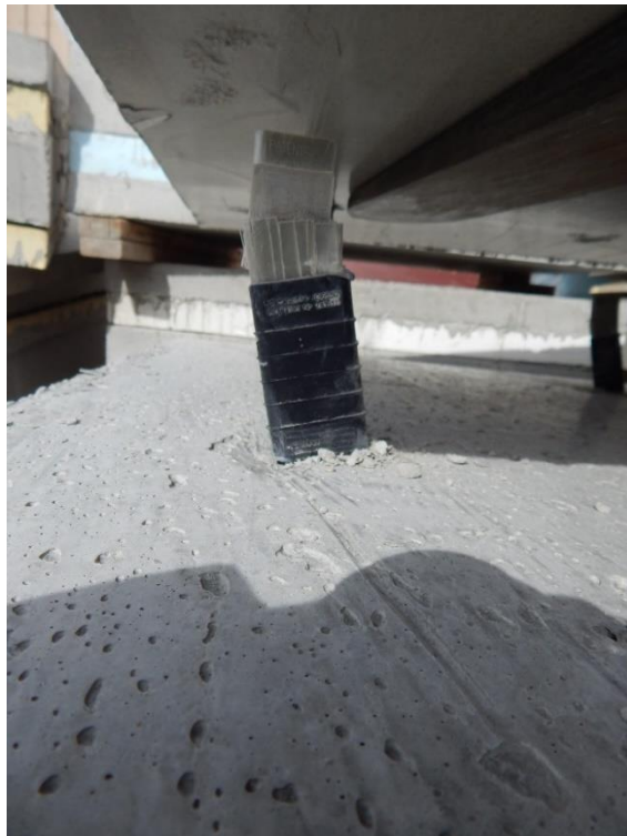
Figure 4-23 Shear fracture observed in Connector B
