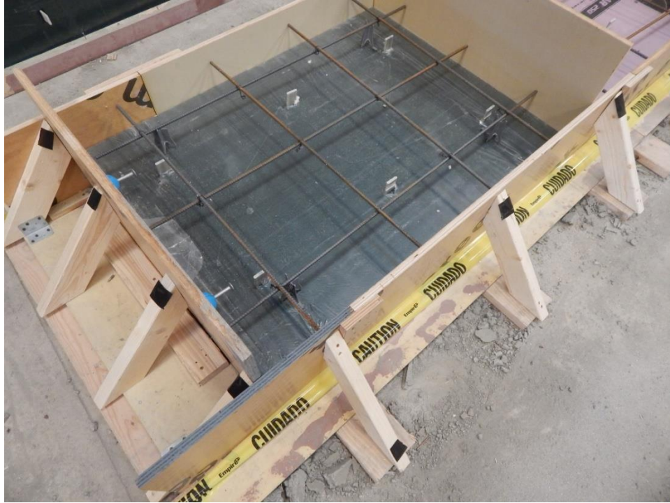
Figure 3-17 Second wythe preparation with rebar, pick-points, and form work in place
