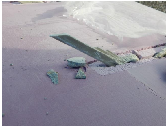
Figure 4-26 Delamination observed in a 4-in. unbonded XPS specimen
