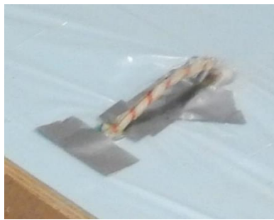
Figure 3-12 Seaming of the bond inhibitor using duct tape
