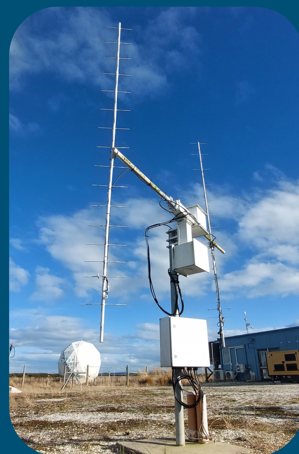
Figure 5 & 6: Measurements provided in this poster were taken on the pictured 400MHz Yagi antenna (AWA-2) and 3.7m S-/X-Band parabolic antenna (AWA-4).
